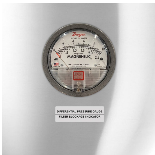
Differential pressure gauge for filter blockage
